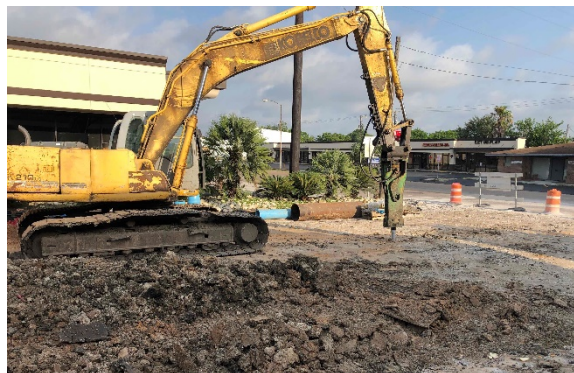
Pavement Demolition on N. Fifth Street
