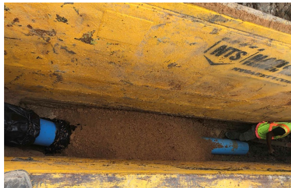
Waterline Installation on N. Fifth Street
