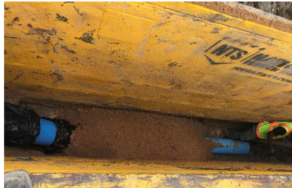
Waterline Installation on N. Fifth Street
