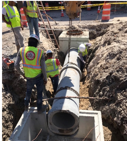
Storm Sewer Pipe & Inlet Installation on Fifth Street
